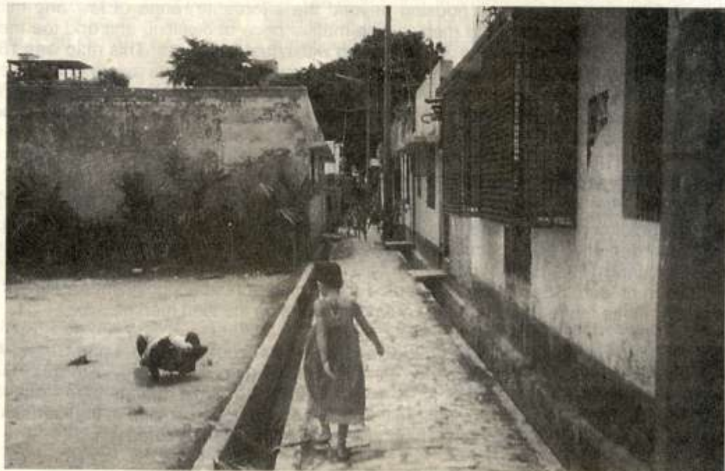
Fig. 1 Plots with infrastructures developed under the Dhaka Urban Infrastructure Improvement Project (DUIIP) at Mirpur, Dhaka.
